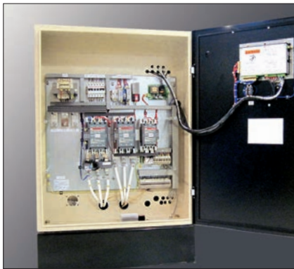
Star delta starter. Soft start is optional.
